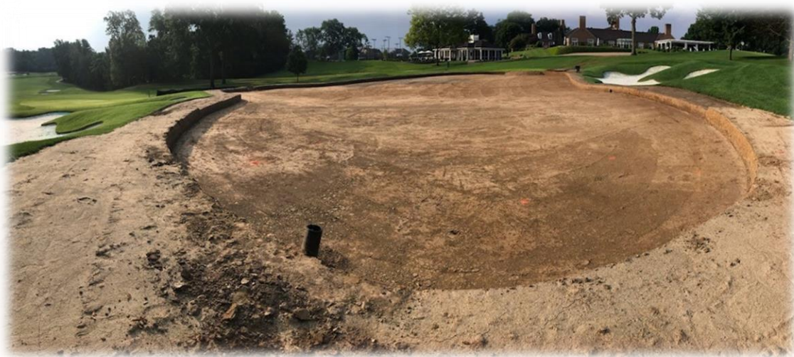
Figure 1-1. Green construction at the Bellerive Country Club (St. Louis, MO)
