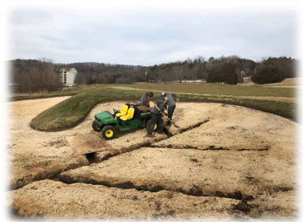
Figure 1-2. Drainage installation at Old Kinderhook Resort, Golf Club, and Spa (Camdenton, MO).
